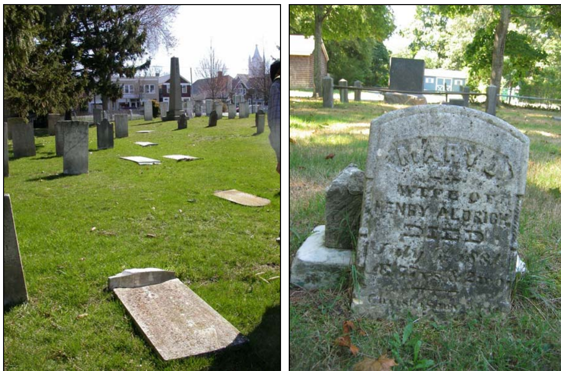
Recent vandalism (April 2004) at North End left a swath of destruction. The older markers were buried deep in the ground and broke just above ground level. Those embedded in bases broke just above the base. To the right, heavy biogrowth on a marble marker under tree cover at East Quogue.
