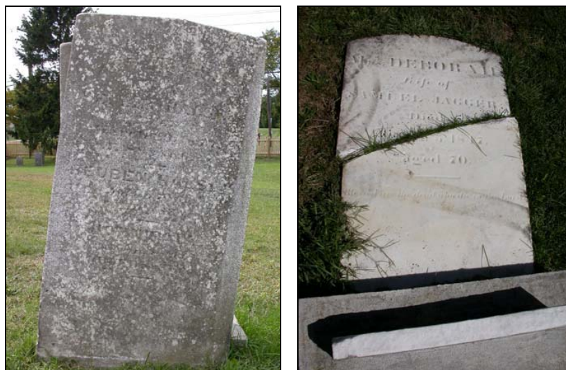
Mold, highly eroded, tilted (left), Recent vandalism breaks (right)
