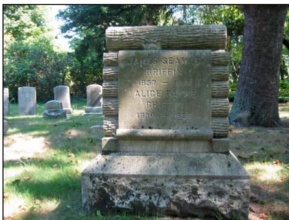
Both at East Quogue, #2066 is an example of cast stone, #2098 is a fine example of the white zinc Pediment styles that were offered through specialized monument companies beginning in the late 1800s.
