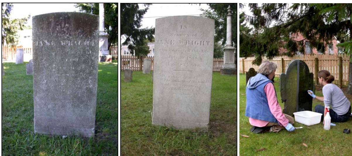
North End Workshop: #031 marble marker before and after cleaning, #119 slate being cleaned.
