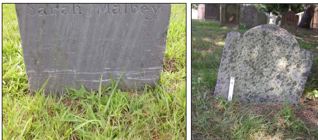
Slate markers: SO2, #726 with mower abrasion and at SO1, #156 is partially buried and badly stained by recent fence ‘clear-coat’ spraying.
